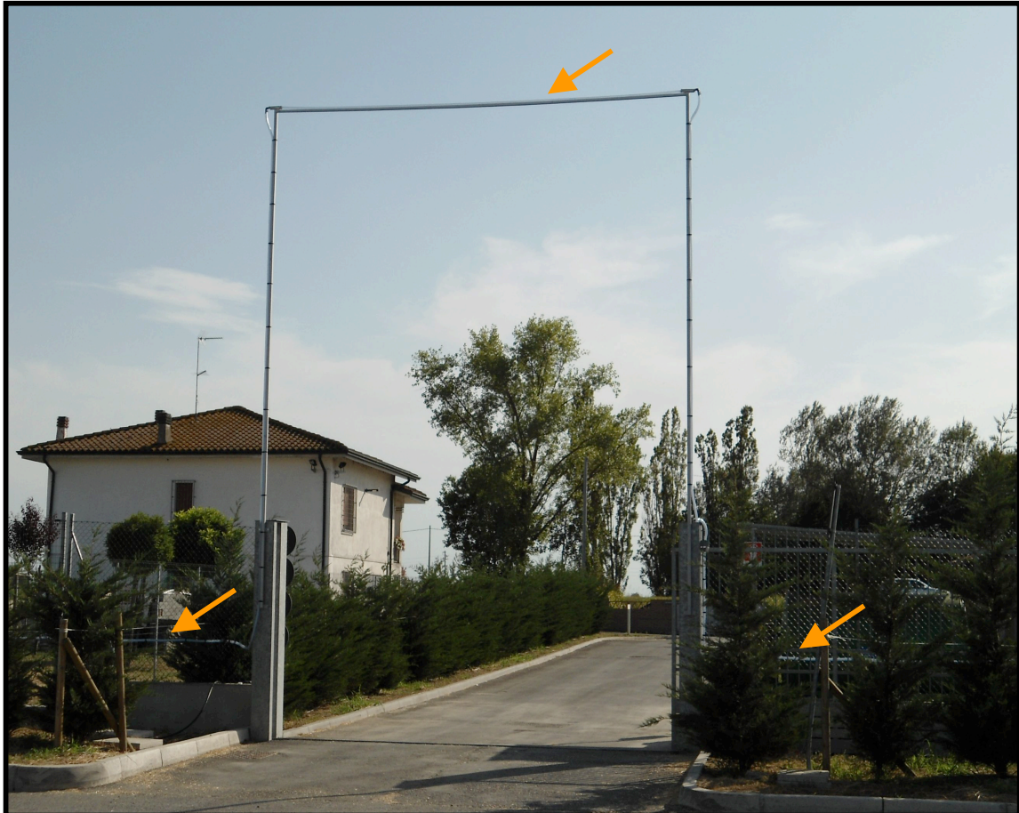
Portico made in the zone 2 place to allow the trucks entrance in the plant:
