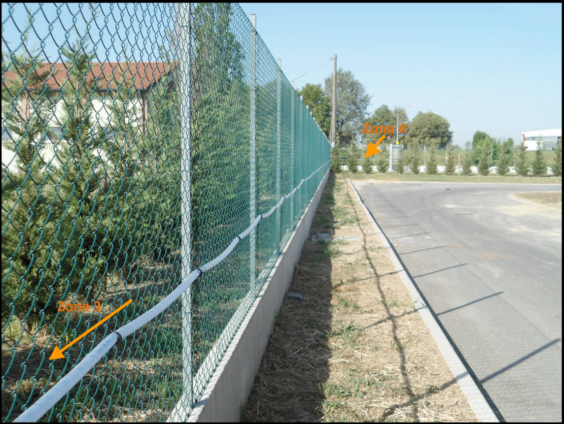
View of the micro-pierced diffusion pipe from the zone 3 to the zone 4:
