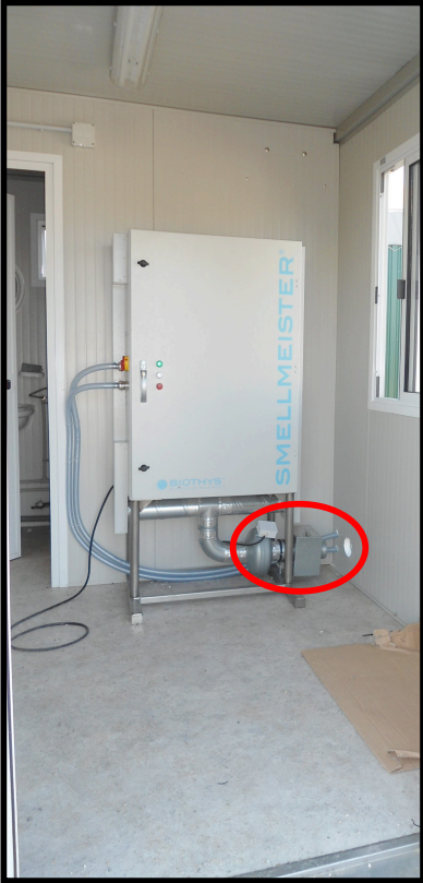
View of the Smellmeister® device installed in the technical room with an external fresh air supply point:
