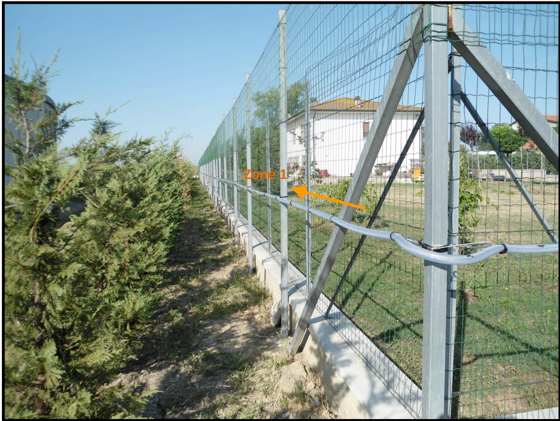
Zone 1 treatment through a micro-pierced diffusion pipe:
