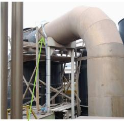
Sheath feeding diffusion ramps inserted in the chimney
